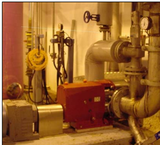
Series S pump in a major soap making plant
