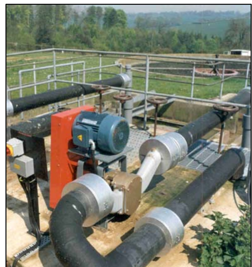
Series D pump on PST De-sludging application
